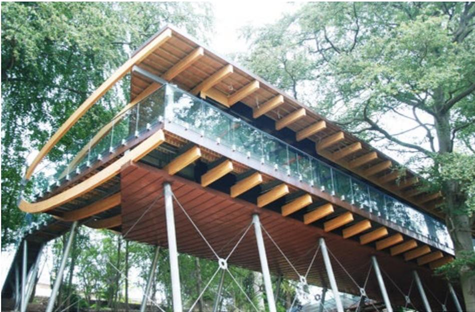
The structure is a simple combination of curved glulam beams encapsulating a space clad in copper, all supported from a steel column and tensile structure below. The wing cantilevers out 30 meters to admire the valley view from some eight meters in the air. A simple yet elegant structure with minimalist materials all designed to age with the surroundings and go some way to putting a local hero finally on the map.
